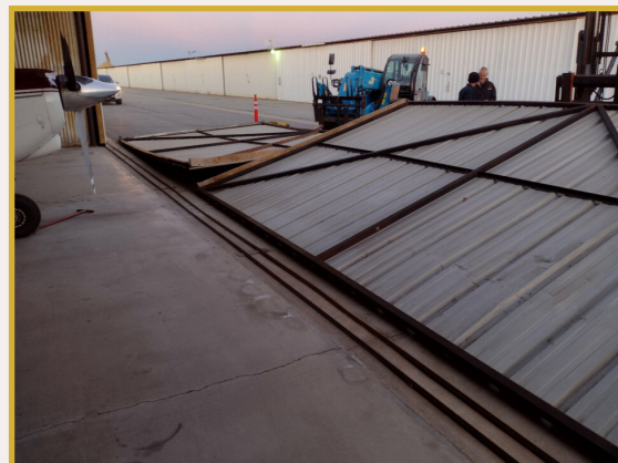
Cable staff reinstalling door that blew down.
